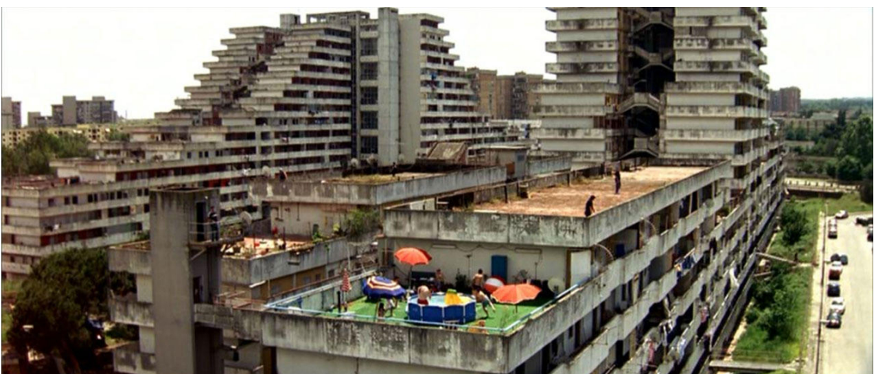
Fig. 7.1: The project buildings “Le Vele” in Sampia (Naples).
