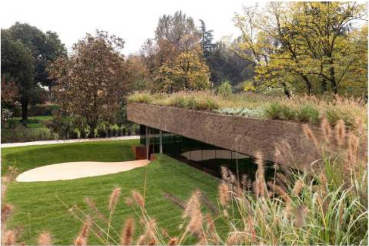
Fig. 2.63 The green roof created from the excavated materials of the construction site allows the building to blend with its natural surroundings. (Agnese Bedini and Melania Della Grave/DSL Studio)
