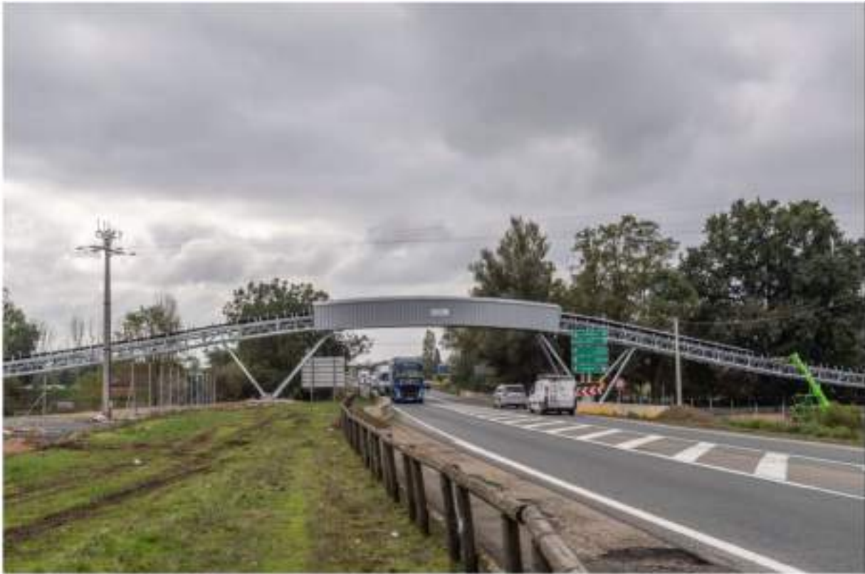
Fig. 2.54 Example of a conveyor crossing a major road
