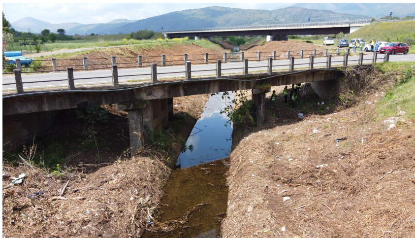
Figure 2.2: Priverno Bridge: Structural context and accessibility.
