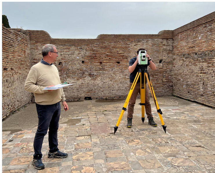
Figure 2.12: Total Station survey for target coordination
