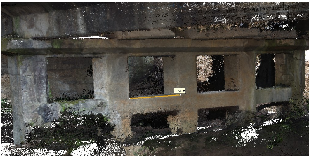
Figure 2.4: Dimensional discrepancy analysis: Digital measure (1.54 m) vs. Real dimension (1.42 m).
