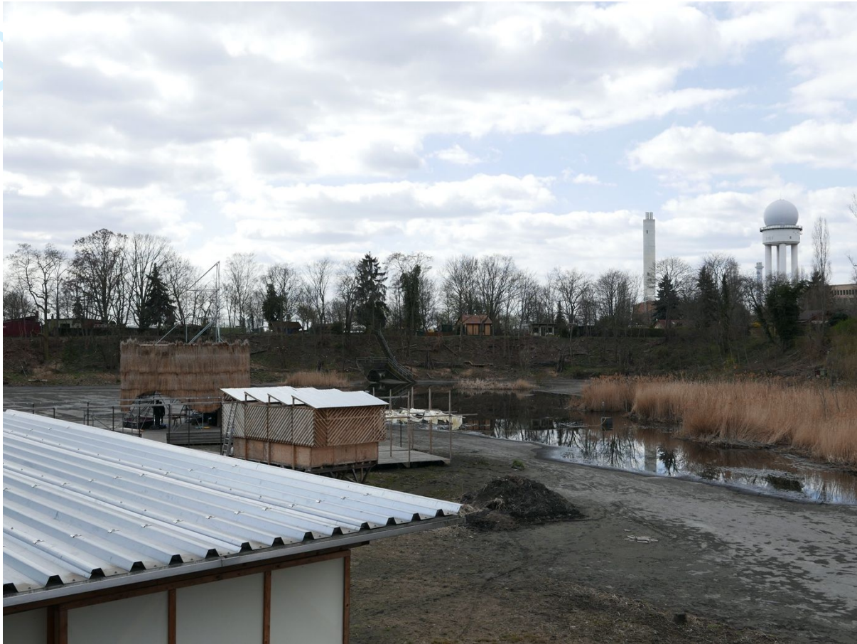
Plate 1. View of the FUB and the detention basin from the entrance. In the background it is possible to glimpse the inlet pipe that gathers the rainwater from the former Tempelhof airport just behind.
