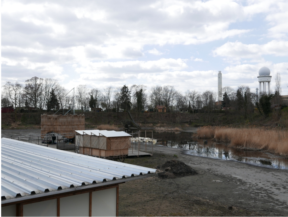
Plate 1. View of the FU and the detention basin from the entrance. On the background it is possible to glimpse the inlet pipe that gathers the rainwater from the former Tempelhof airport just behind. Photo credits: Federico Brogini
