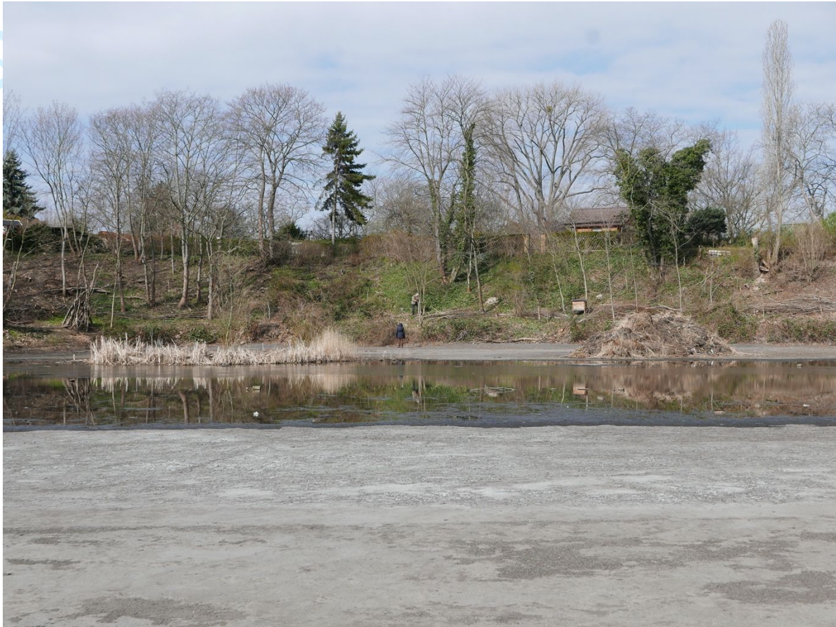
Plate 2. View of the slope forming the detention basin. The photo shows a phase of vegetation maintenance, in particular the pruning of trees.
