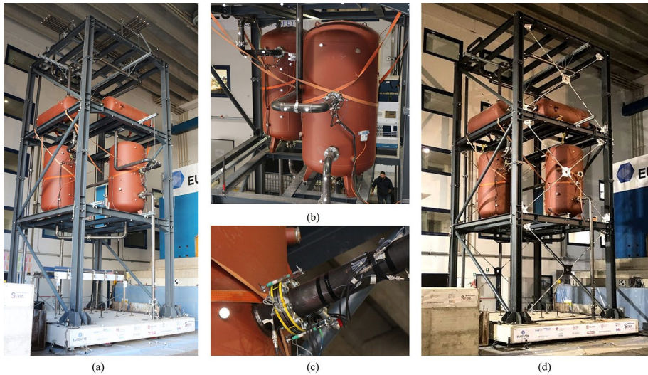
Fig. 1 Photos of the SPIF's mock-up tested in EUCENTRE lab, Pavia, Italy: a the MRF configuration; b the two installed vertical tanks; c details of the BFJ between the vertical tank and the piping system at 1st level; d the BF configuration
