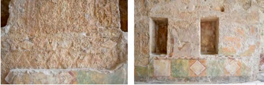
Fig. 9.4 Left: detail of the rustic mosaic warp—right: right wall of the Nymphaeum, painted plaster imitating marble slabs
