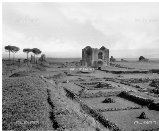
Fig. 1 - View of the Mausoleum of Sant'Urbano on Via Appia Antica in Rome, around 1910 (Archivi Alinari, Florence).
