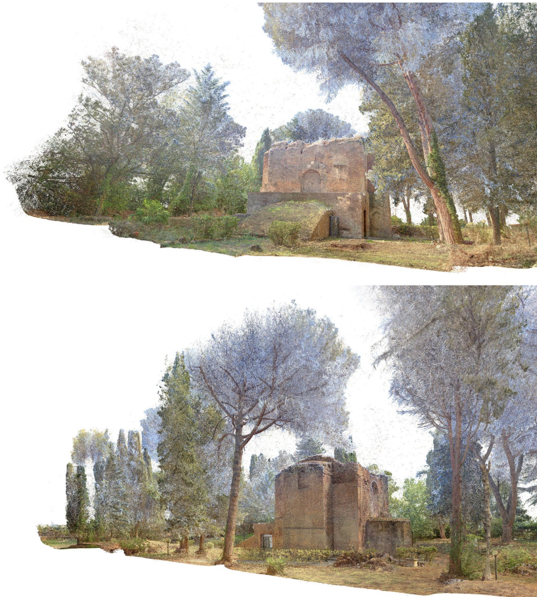
Fig. 8 - Screenshot of the point cloud of the site: the main facade (graphic elaboration by the authors).
