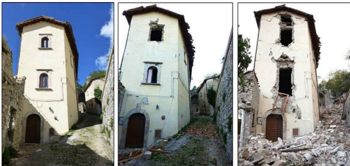
Figure 23. Example of the effects of damage progression in a class B building in Castelsantangelo sul Nera: left) August 24; center) October 26; right) October 30 [from Rossi et al., 2019].
