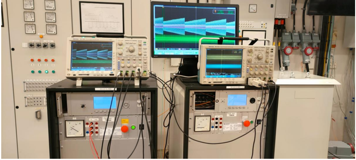
Figure 74 - Test setup for measuring the three-phase currents and voltages directly calculated by the FPGA.
