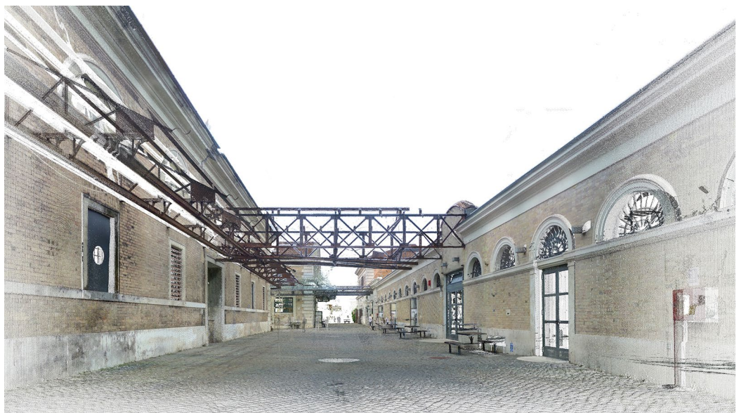
Fig. 5. View of the point cloud of the ex Mattatoio. On the right, it is possible to notice artifacts caused by the reflections of the windows and, on the left, some blind areas caused by the metal structure. Graphic elaboration by the authors.
