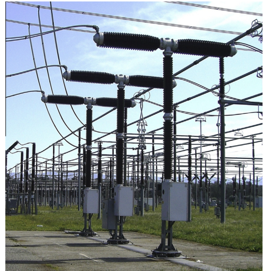
Fig. 21. Installation of the seismic isolation system.
