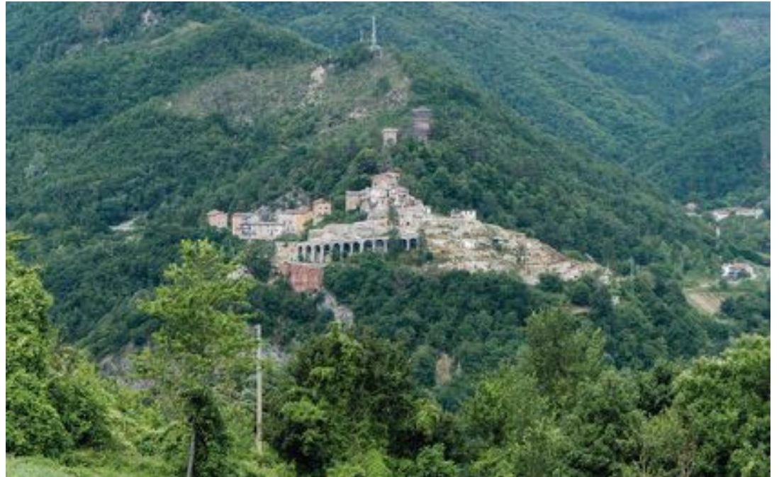
Fig. 1. A view of the destroyed village of Arquata del Tronto.
