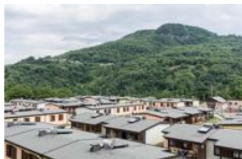
Fig. 2. The temporary SAE camp in Borgo, Arquata del Tronto near Ascoli Piceno (photo credits: A. Gabbianelli).
