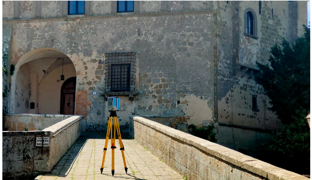
Figure 5. Photo taken during the survey campaign, showing the laser scanner employed and one of the targets located on the wall next to the entrance arch. Different quality levels were used during the scanning process, mainly based on the distance between the artifact and the device. In particular, external scans were set to a higher-resolution quality to obtain greater accuracy of the data (image by the authors).
